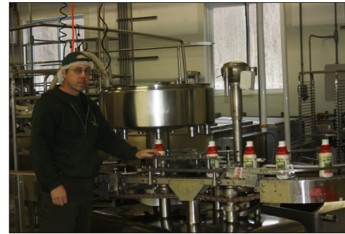
Bob Yaroshevich of Y Enterprises installing new bottling equipment at Vermont Soy in Hardwick.
